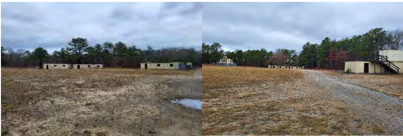
Figure 3: NBC Open ground and conex buildings
