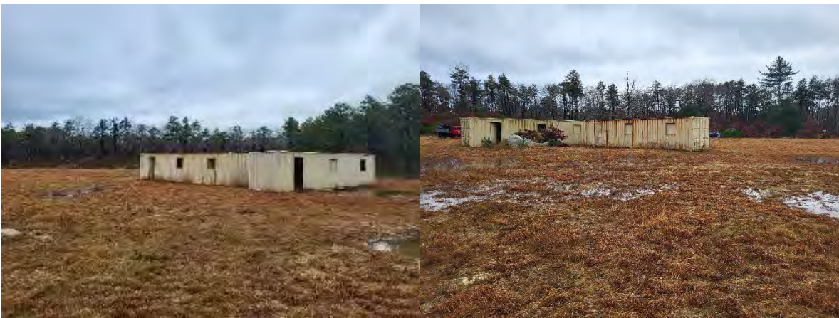
Figure 6: BP 24 Showing front (left) and back (right) of conex buildings
