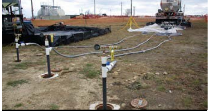
In-situ chemical oxidation operation
